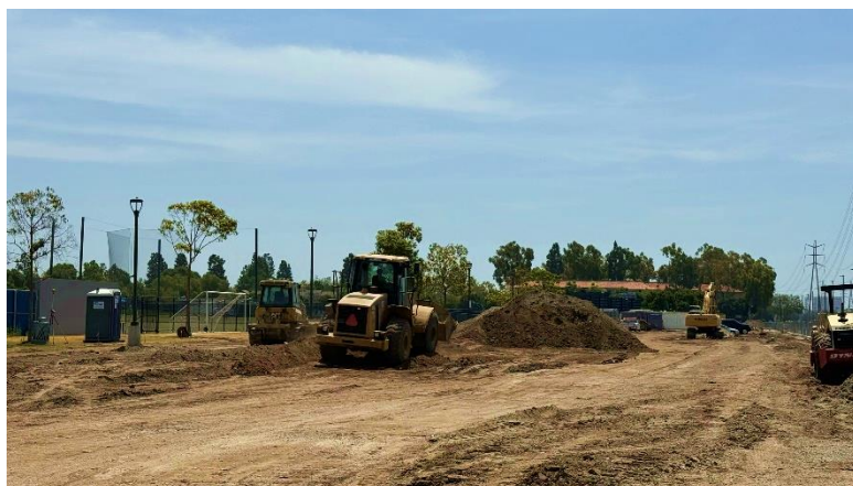
Parking Lot Grading – West Elevation
