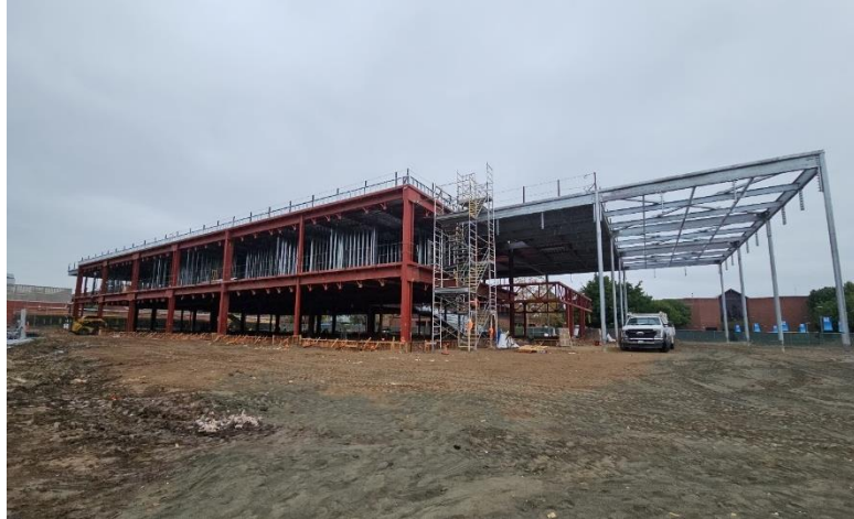
Student Service Center – North Elevation
