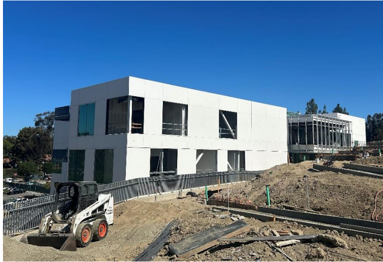
Math and Computer Science Building – Southeast Elevation
