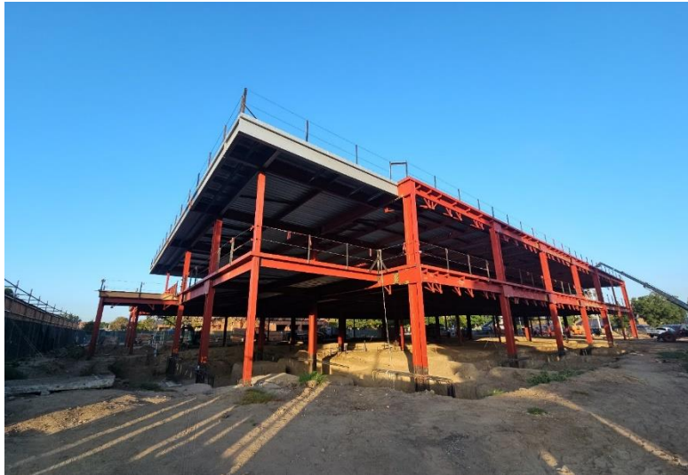
Student Services Center – Northeast Elevation
