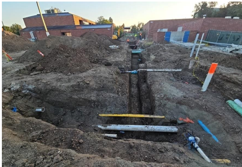
Student Union Utility Work – North Elevation
