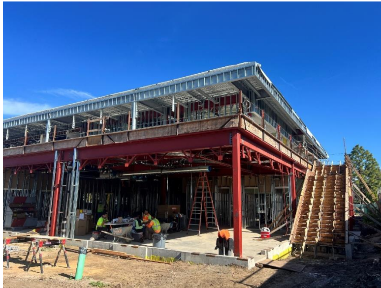
Student Services Center – Southwest Elevation
