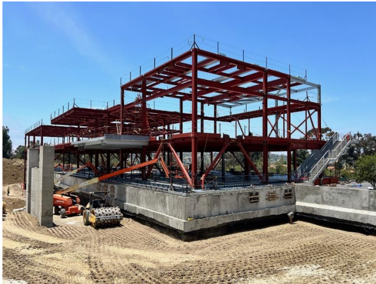
Main Retaining Wall – Northeast Elevation
