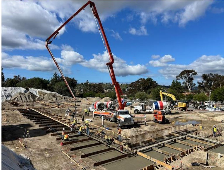
Retaining Wall Foundation – North Elevation
