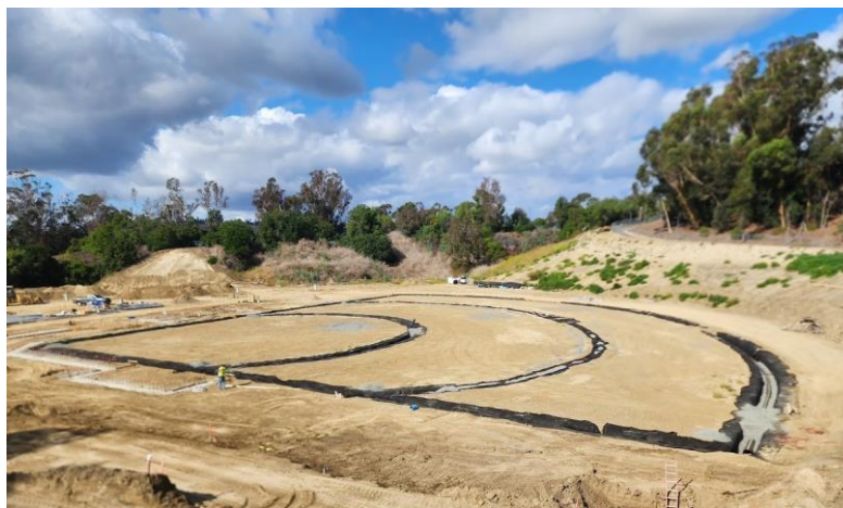
Softball Field Drainage – Southeast Elevation
