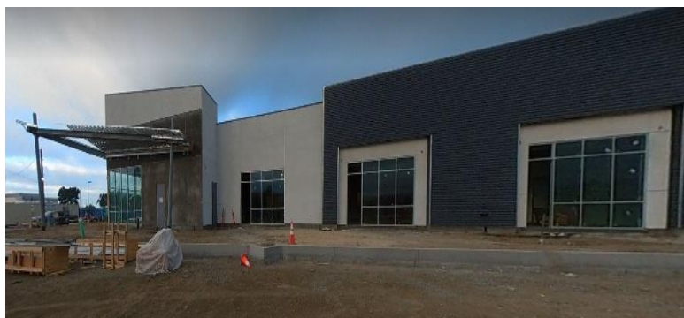
Goddard School Building – East Elevation
