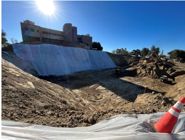
Building Grading – East Elevation
