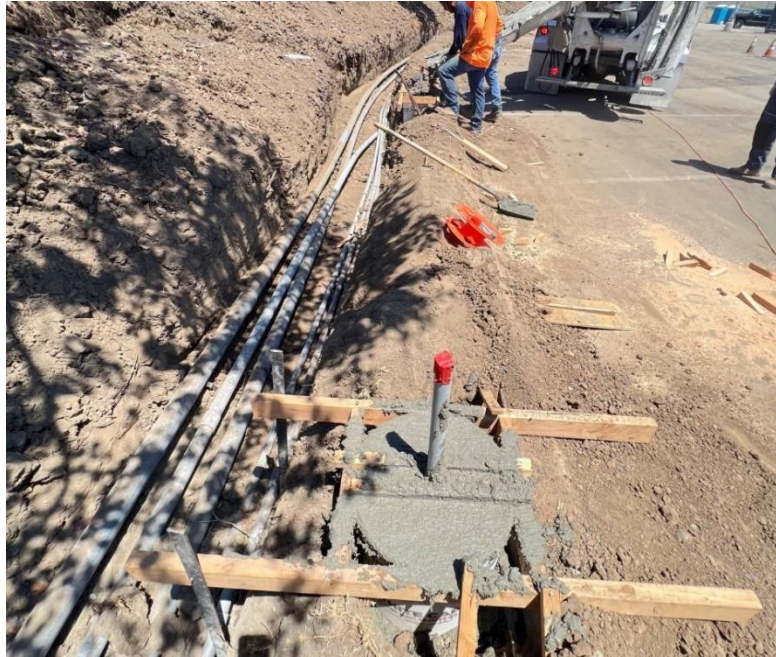
EV Charger Footings
