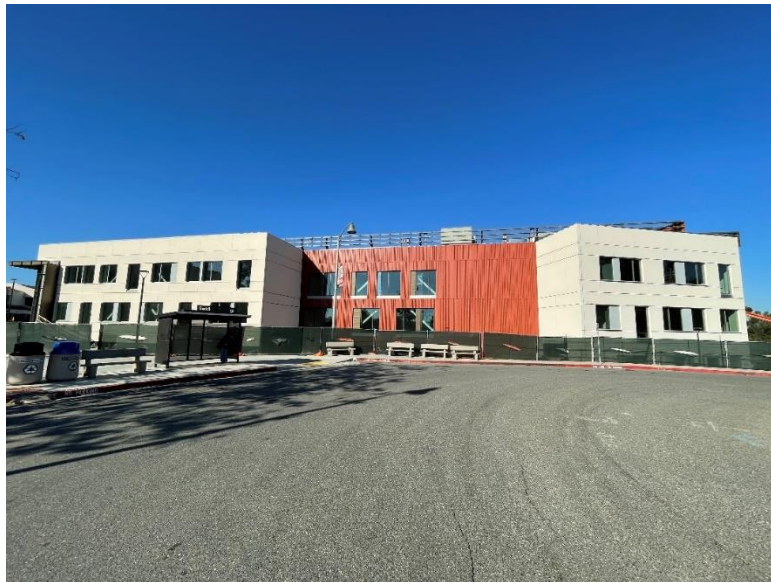
Medical Center Drive Entrance – Northwest Elevation
