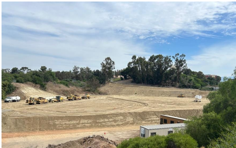
Site Grading – South Elevation
