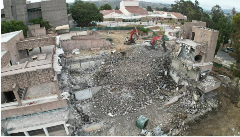
South Section Demolition
