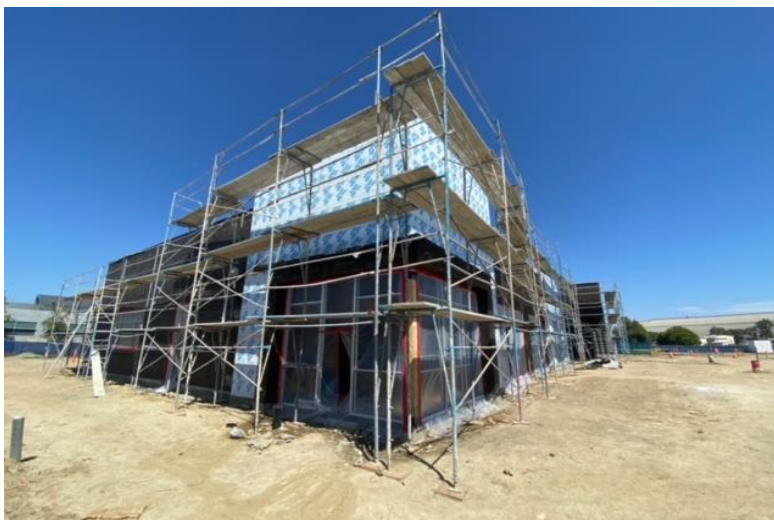
Building Framing – Southwest Elevation
