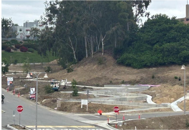
ADA Pathway at Medical Center Drive Entrance
