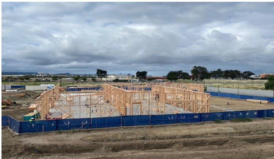
Building Framing – North Elevation
