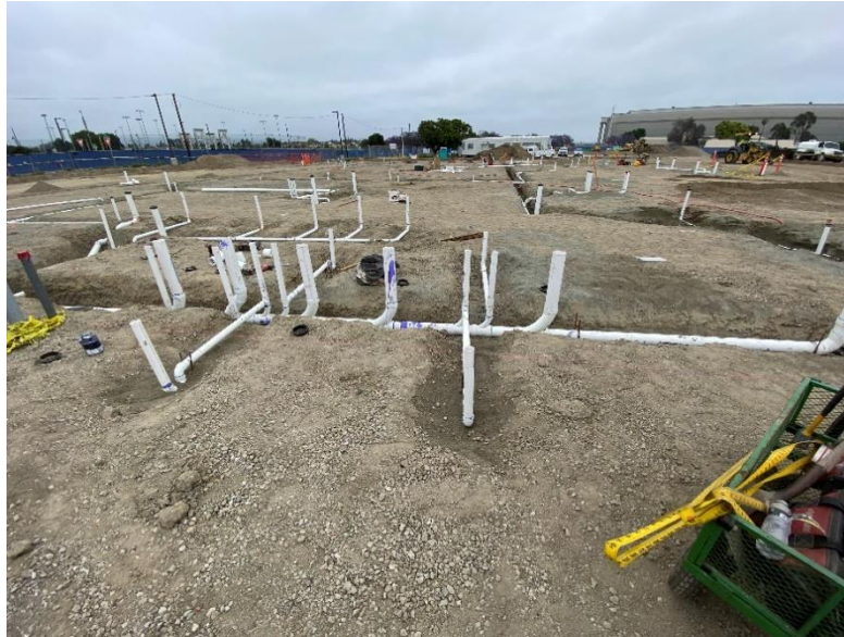
Underground Plumbing – West Elevation
