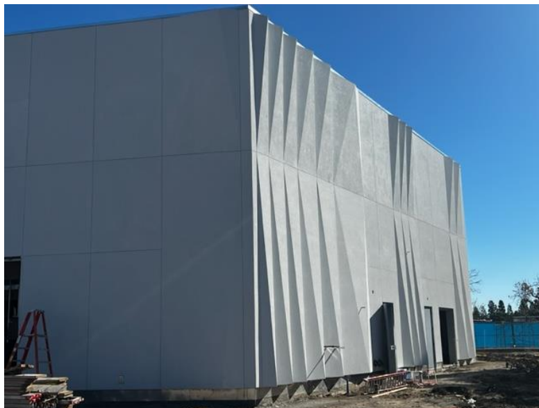
C Building – West Elevation
