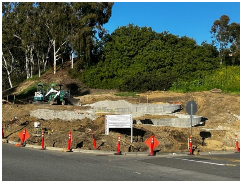
Retaining Walls at ADA Pathway at Medical Center Drive Entrance
