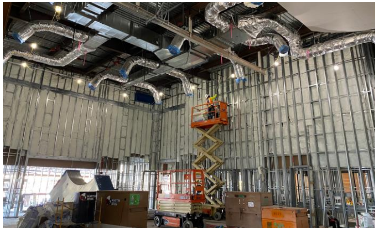
Lecture Hall Interior Framing and Ductwork
