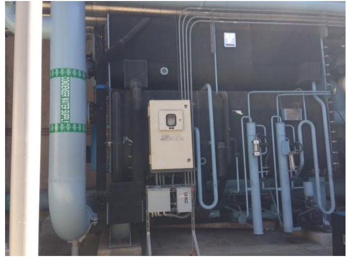
Central Plant Absorption Chillers
