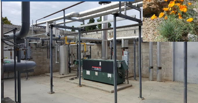
Replacement of antiquated boilers with new energy efficient models
