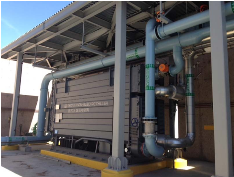
Central Plant Absorption Chillers
