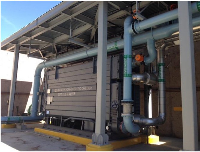
Central Plant Absorption Chillers
