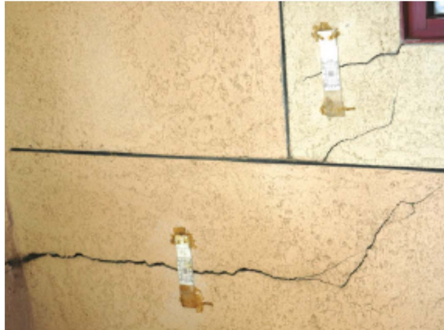
Monitoring crack separation
