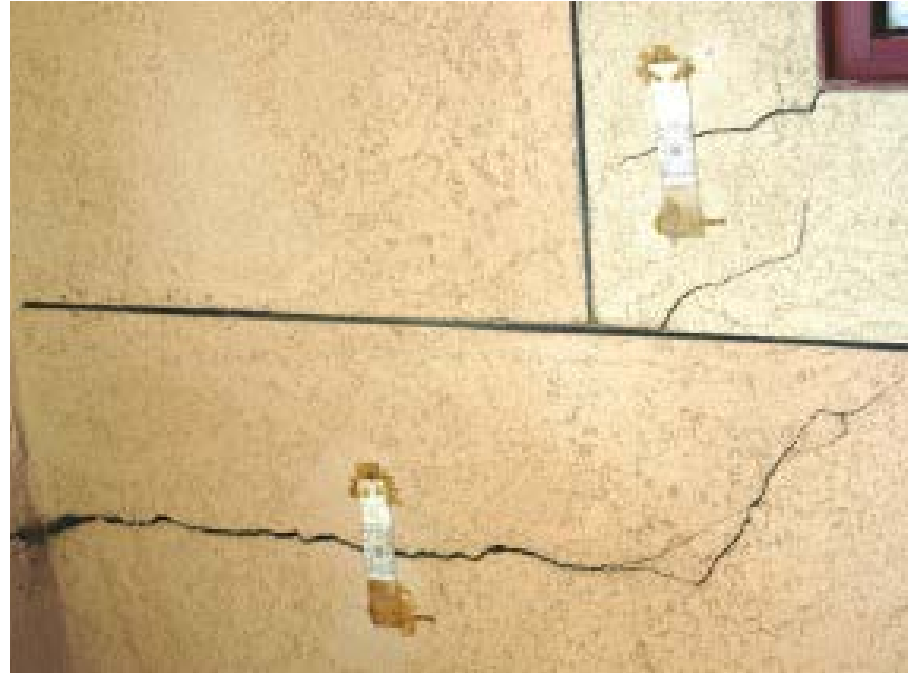
Monitoring crack separation
