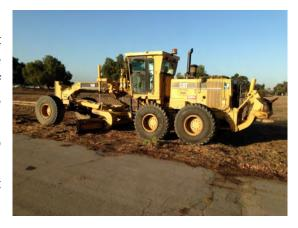
Graders are now completing rough grading of the site to promote good storm drainage and runoff while also providing a smooth surface for easy care and mowing of the new hydro-seeded natural grasses.
