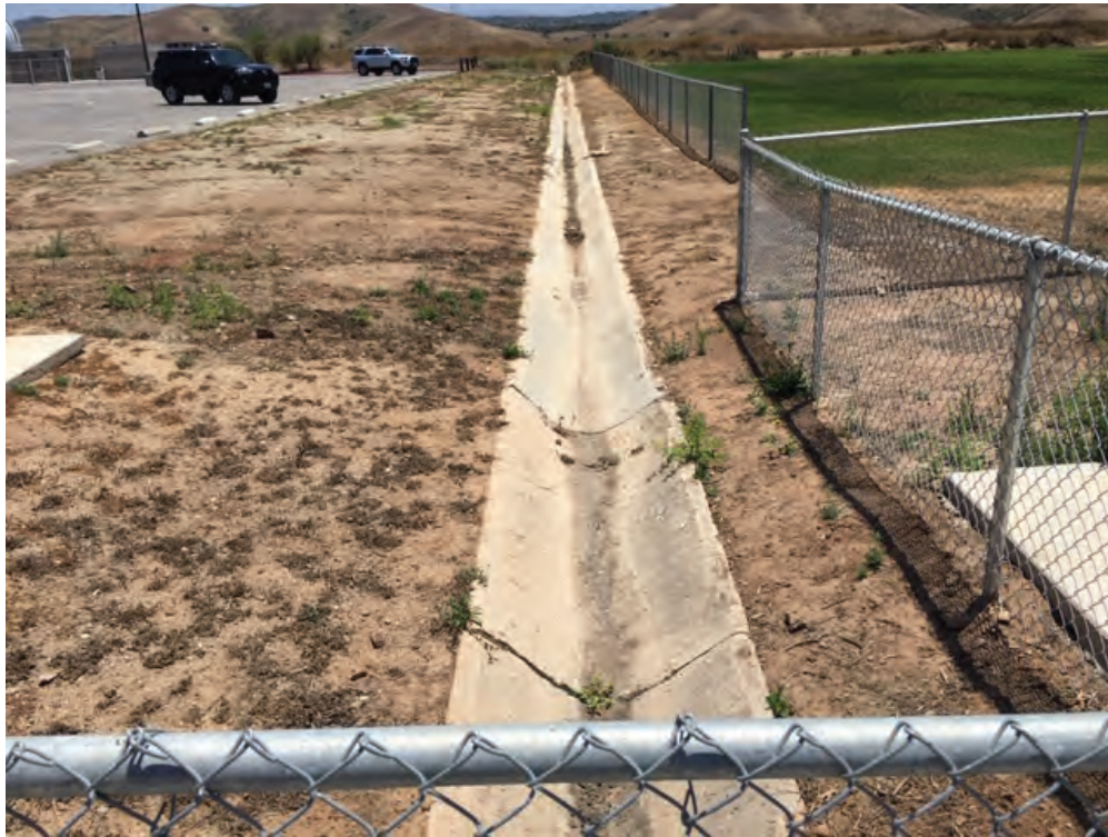
Photograph 5: Brow ditch across the northern portion of the Project site.
