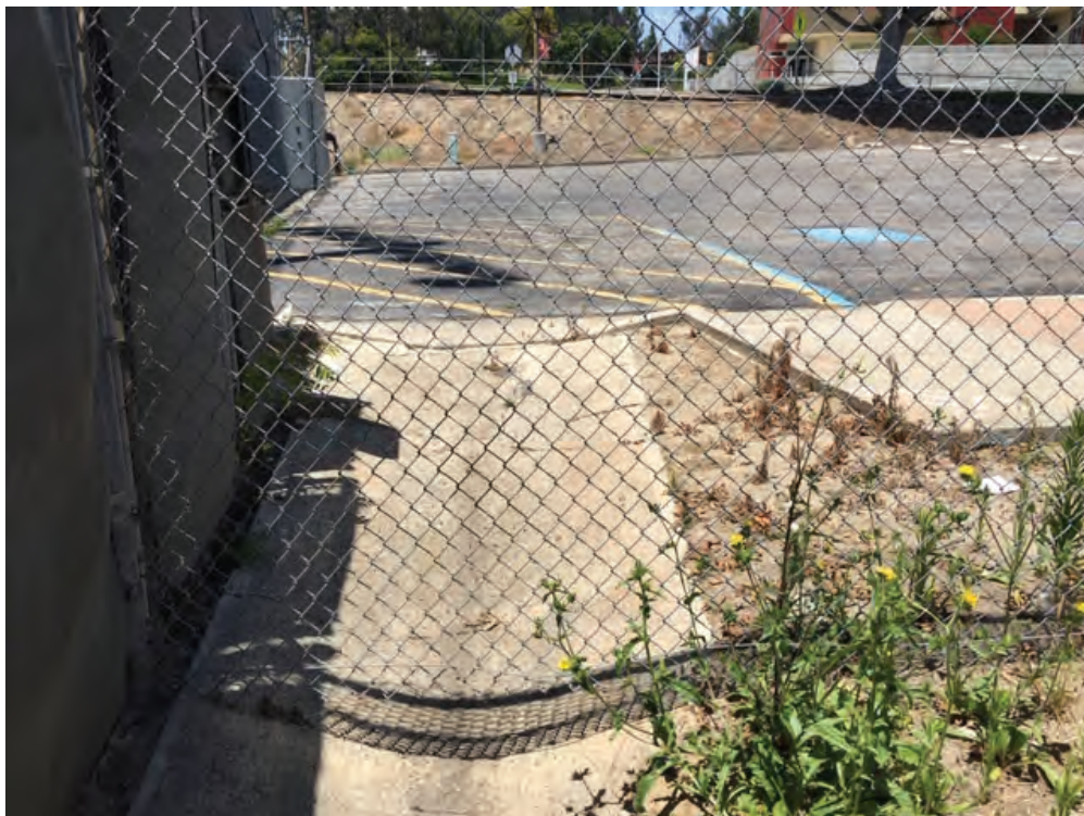
Photograph 2: Origin of the southern brow ditch at the parking lot edge.
