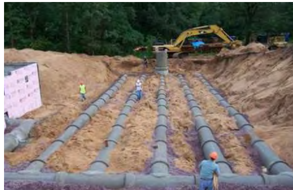
Earth Tube Section
