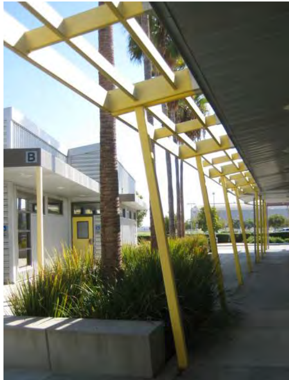
Shade structure. ATEP original facilities
