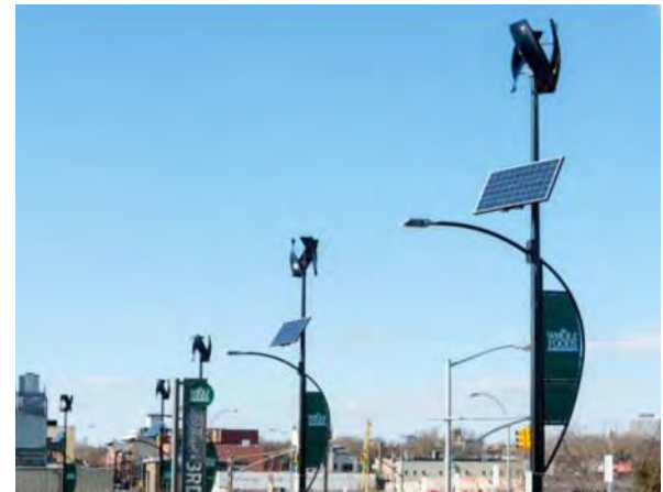
Hybrid Wind/PV street lighting, source: urbangreenenergy.com
