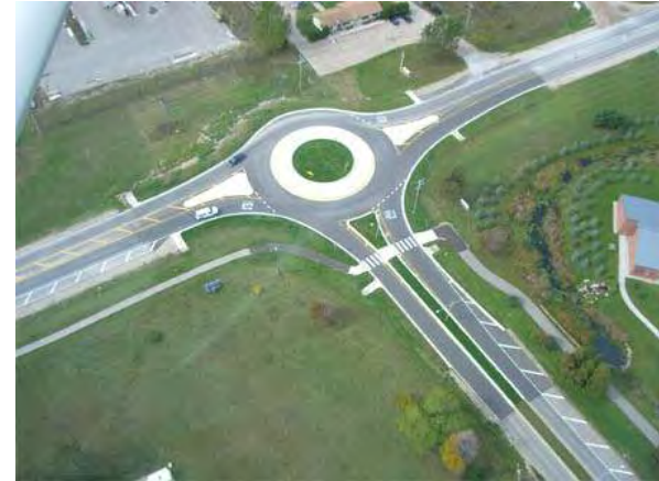
Roundabout with splitter islands
