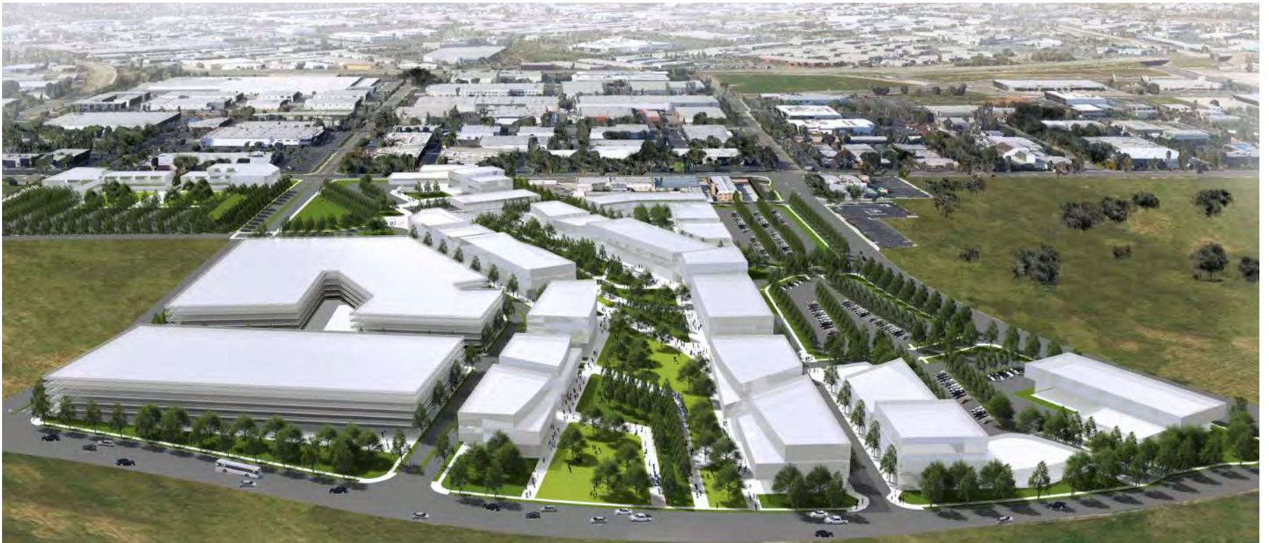
AERIAL VIEW FROM THE SOUTHEAST, LOOKING TOWARD THE NORTHWEST
