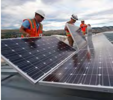
Photovoltaic panels installation
