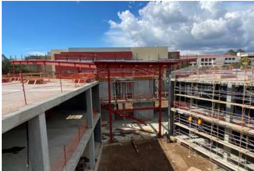
ATAS Building – East Elevation
