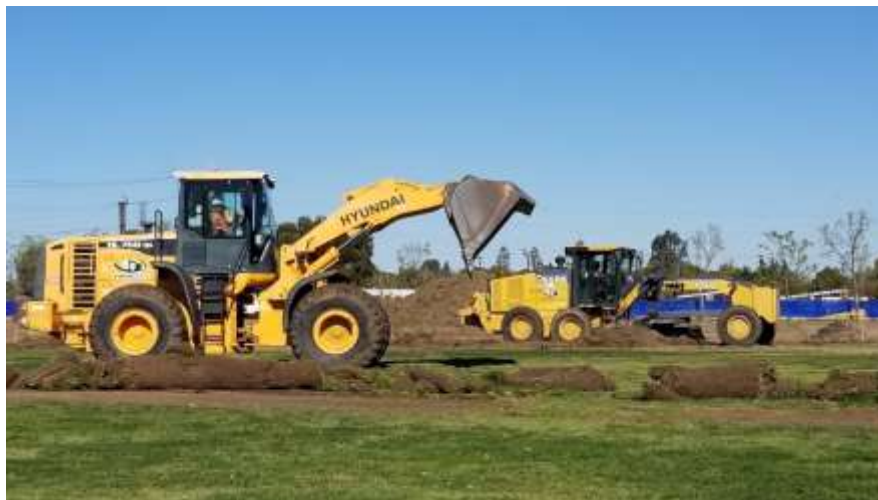
Removal of Existing Turf and Beginning Rough Grading of Soccer Fields
