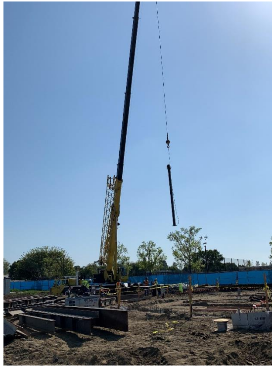
Building C – Structural Steel Erection Begins
