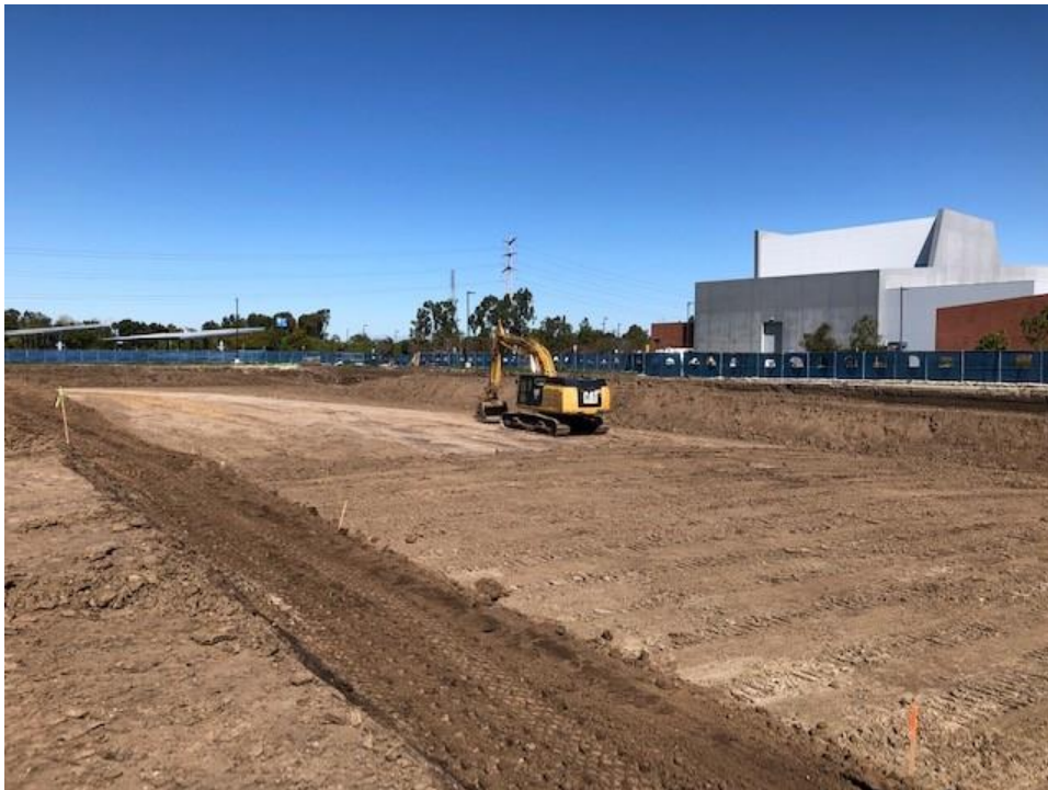
Building A – Over-Excavation Continues
