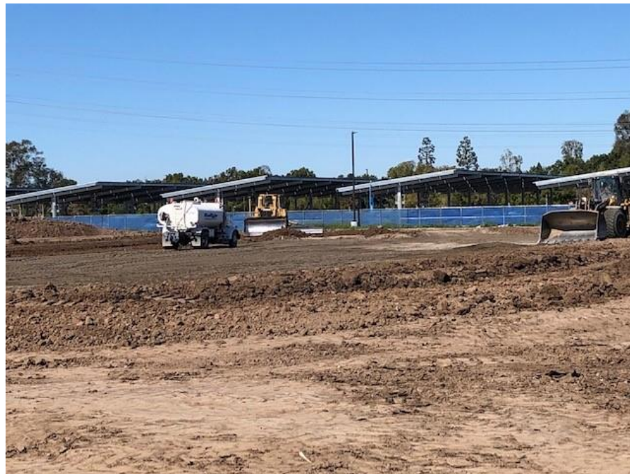
Building B – Backfilling Operations
