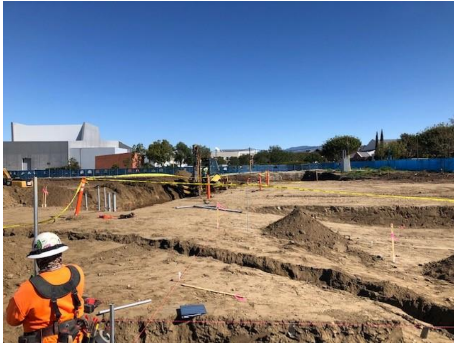
Building C – Starting Footing Excavation
