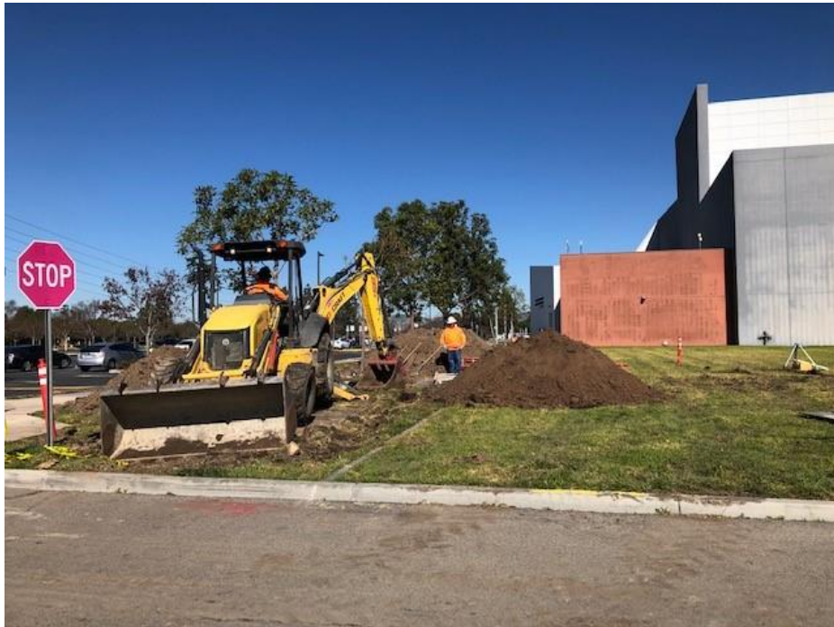
Potholing for Sewer - NW corner 02-07-22
