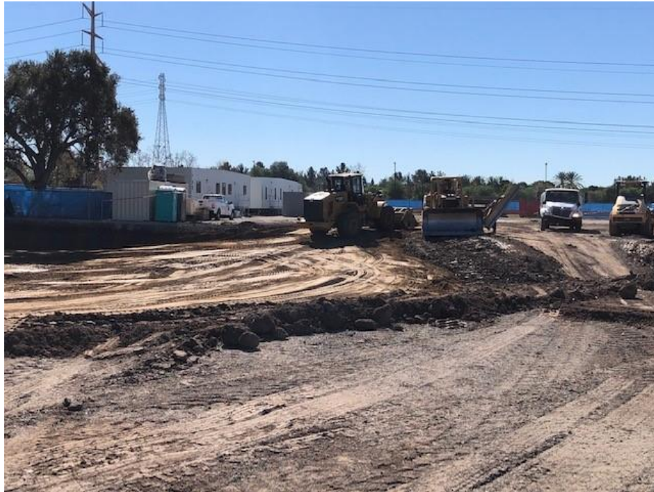
Building C – Completing Import Soil up to Building Pad
