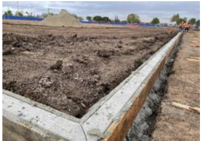
Poured Inside Curb at the Varsity Soccer Fields
