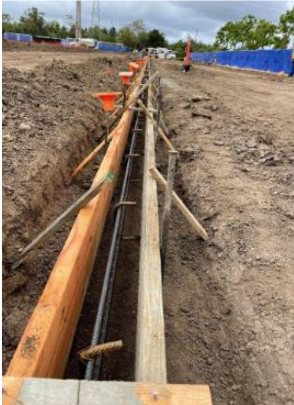
Forming Inside Curb at the Varsity Soccer Fields
