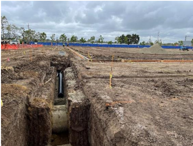
Storm Drain Piping Installation at Existing 30" Main
