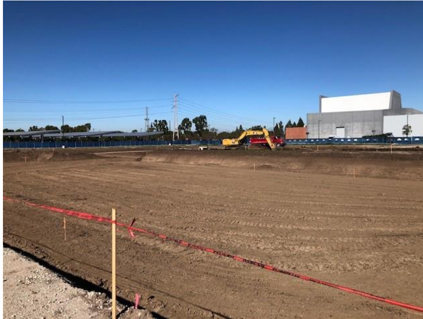
Building B - Building Pad Excavation
