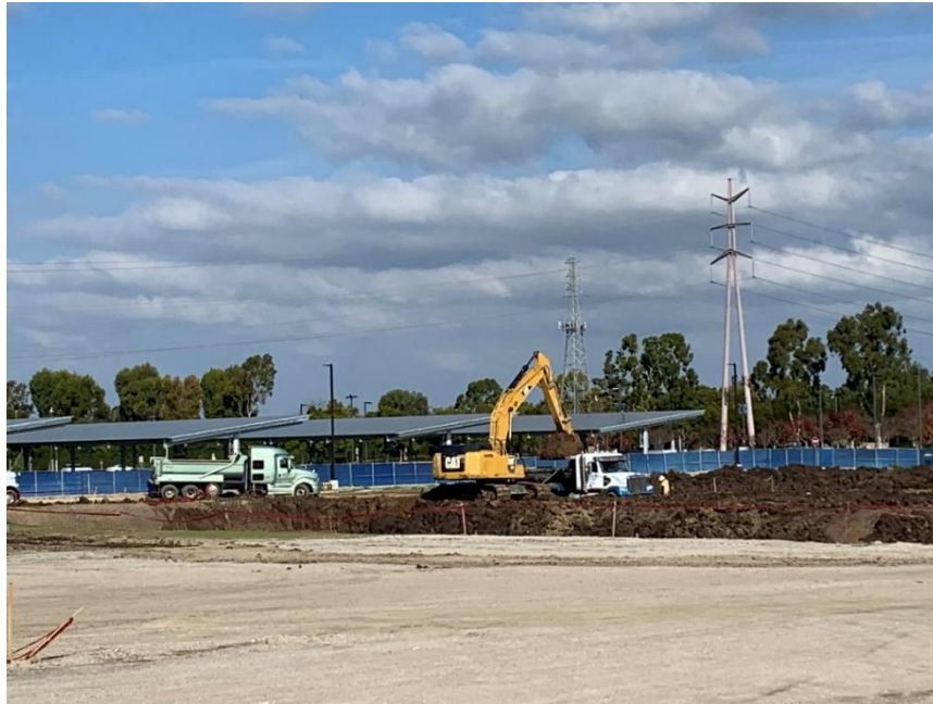
Building A - Building Pad Excavation
