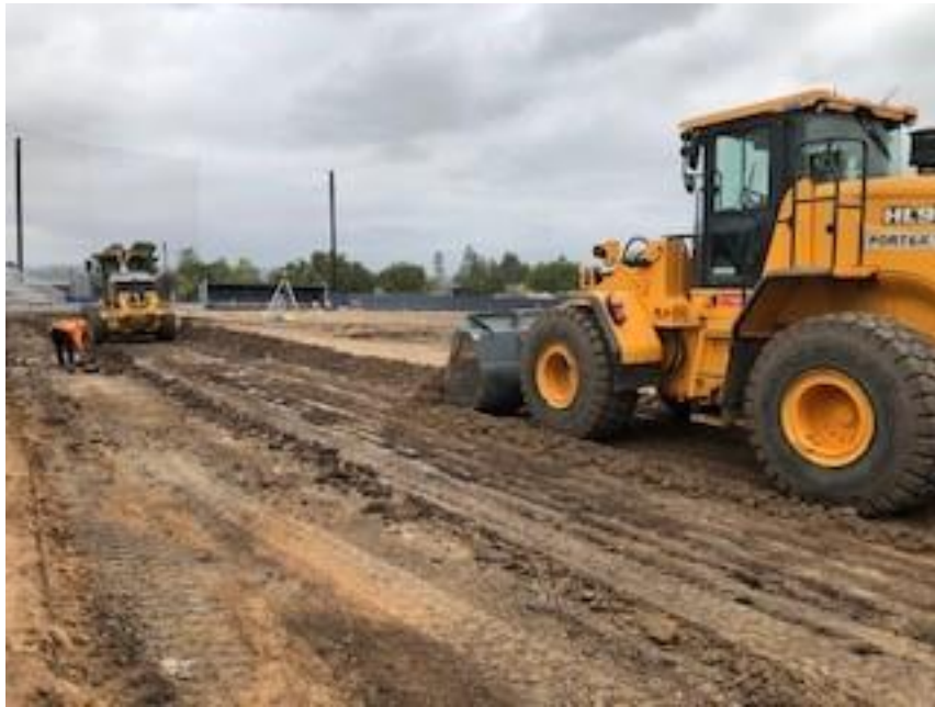
Grading Operations at the Baseball Field
