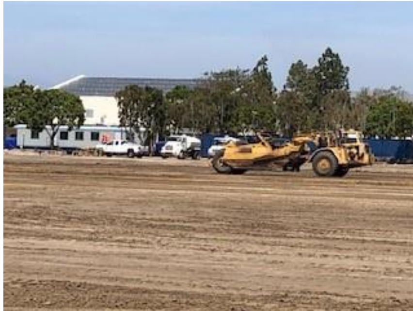
Grading Operations at the Soccer Fields
