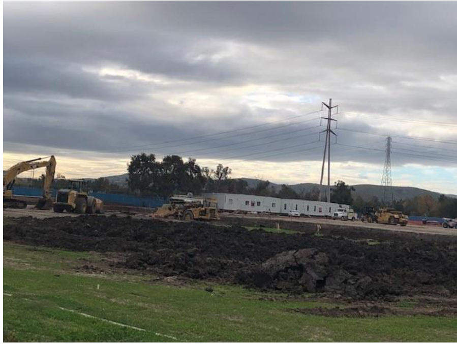
Building B Building Pad Excavation
