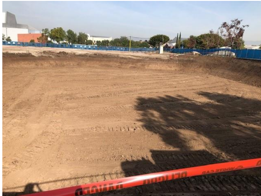
Building B Building Pad Excavation
