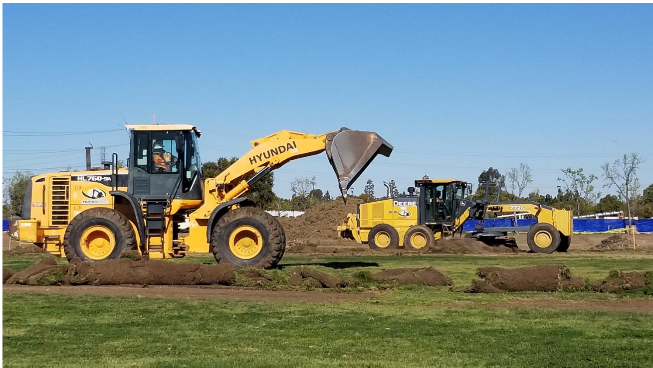
Existing Turf Removal
