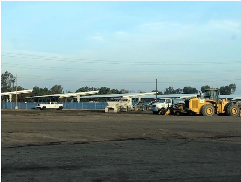
Trucking Exporting Soils from Building B Excavation
