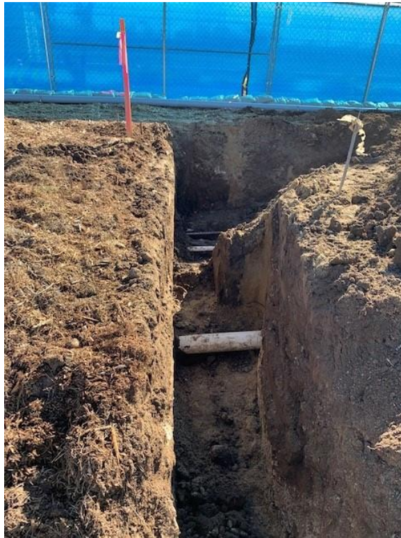
Potholing for existing lines
