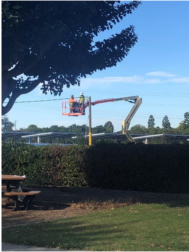
Installation of Temporary Power Poles
