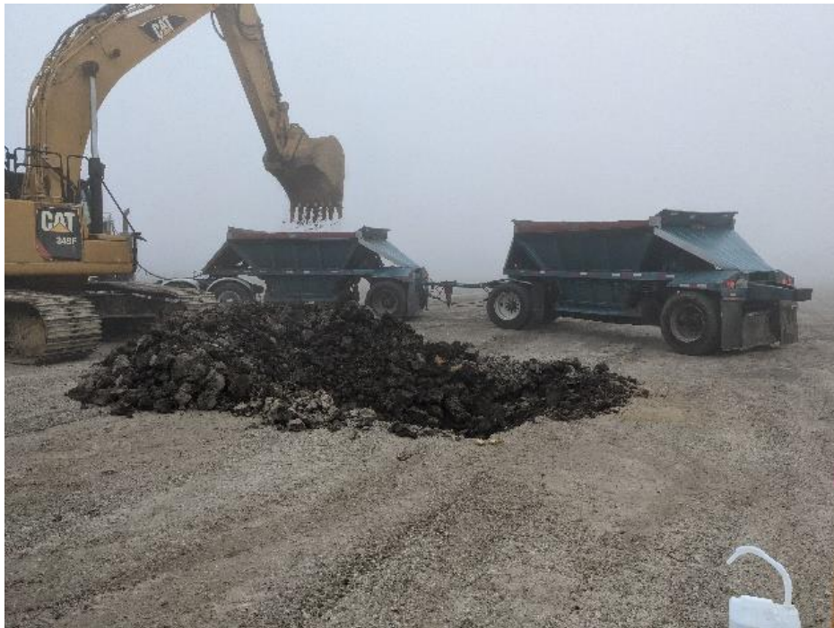
Starting excavation activities
