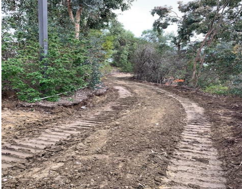
SC Fine Arts Area 5 – Concrete Removed and Preparing for Concrete Installation
