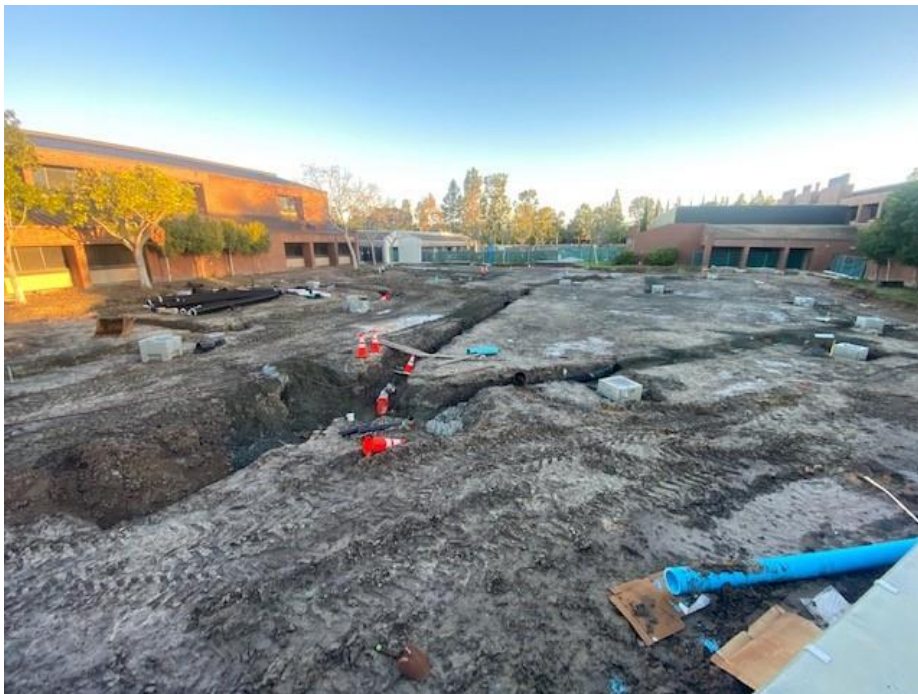
IVC B Quad – Site Overview with New Trenches for Storm System and Storm System Connection
