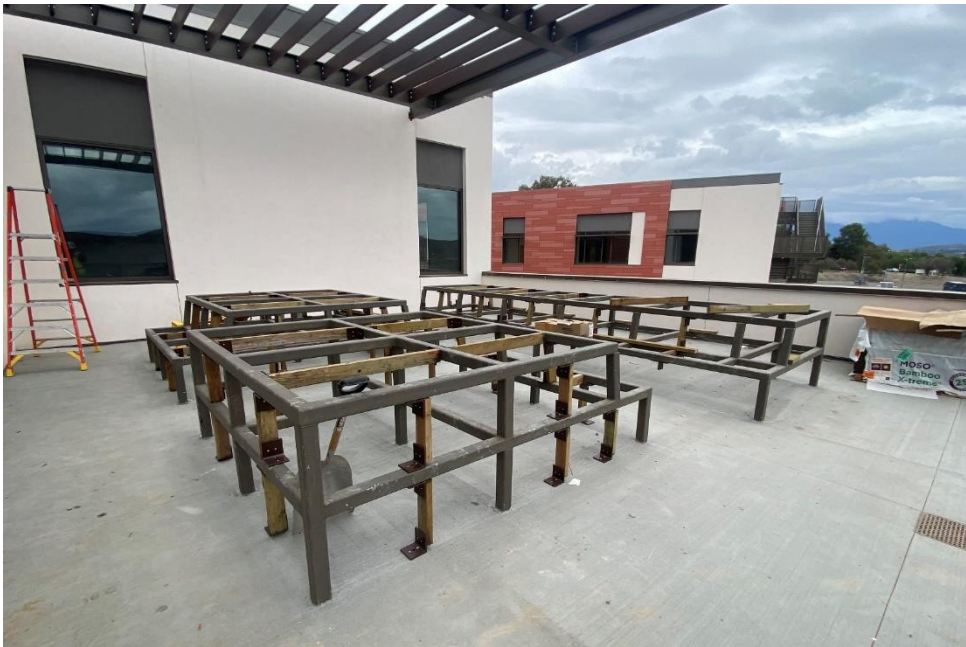
South Wing Outdoor Patio
