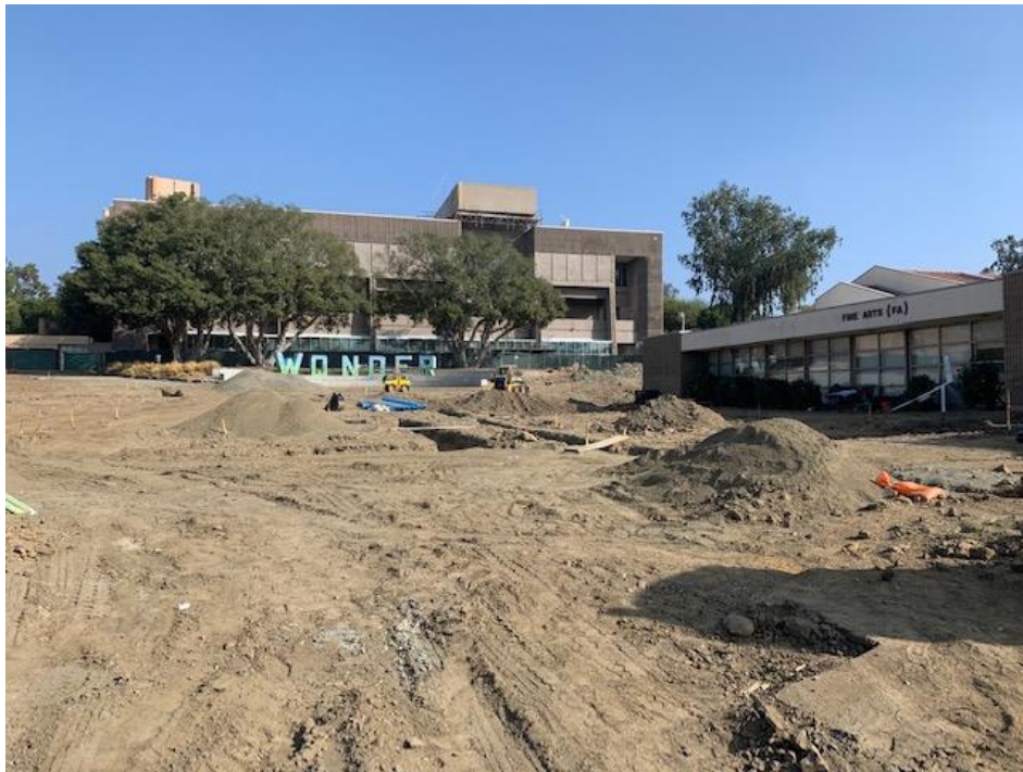
Saddleback College Fine Arts Quad Area – Site Grading and Storm/Sewer Installation
