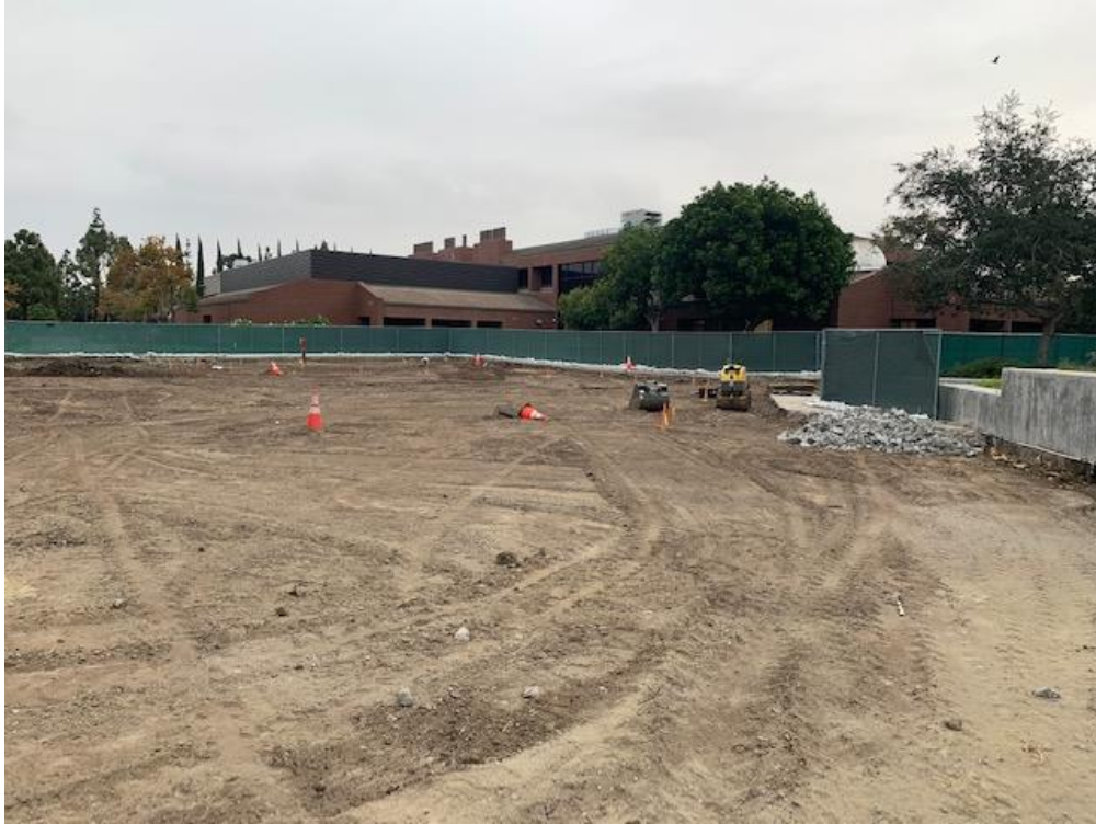
IVC B Quad – Grading and Demolition of Site Concrete at Irvine Valley B Quad
