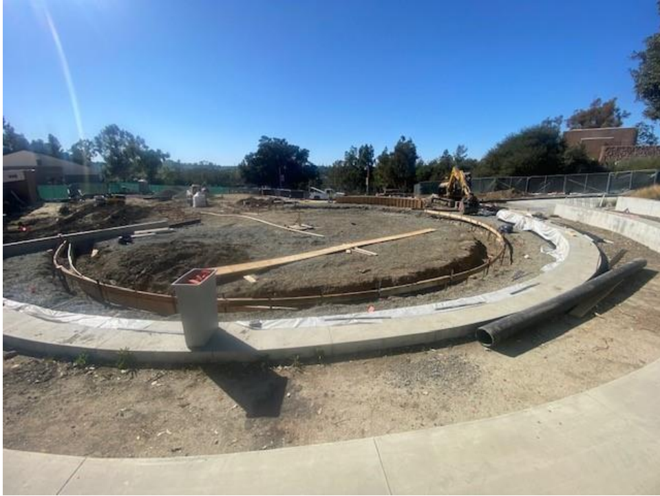
SC Area 5 – Framework Installation in Fine Arts Quad
