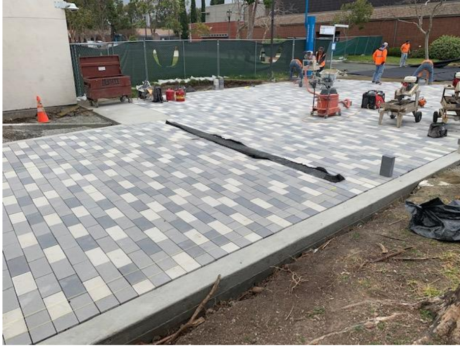
IVC B Quad – Installation of Pavers at IVC B Quad Area
