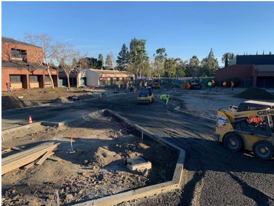
IVC B Quad – Concrete Paving Bands Installed and Base Compacted
