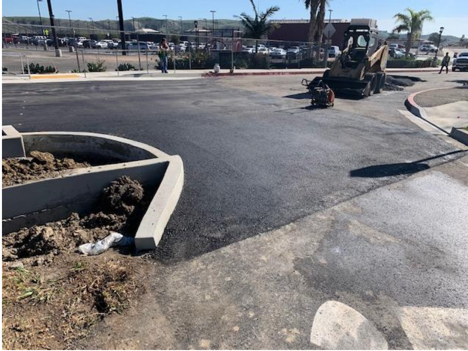
SC Area 5 (College Drive) – Asphalt Paving for ADA Crosswalk between Area 5 & 6
