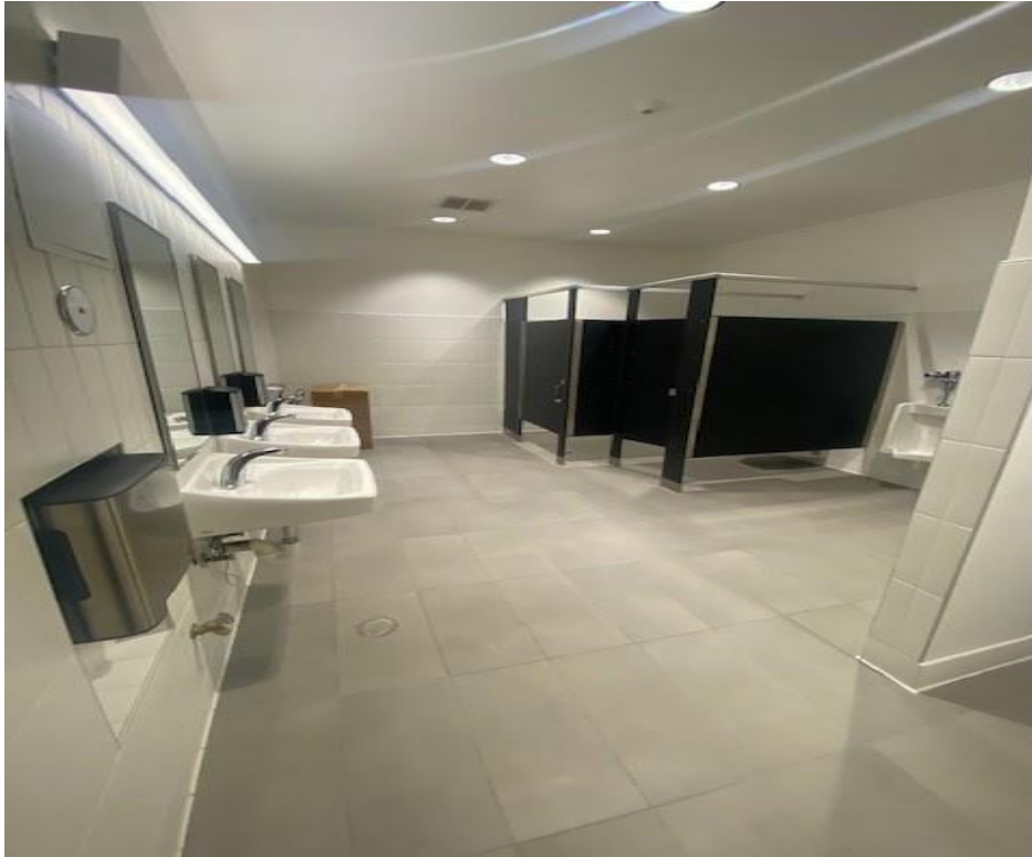
IVC A200 Restroom – Toilet Accessories Installed and Newly Installed Lighting Fixtures Illuminated
