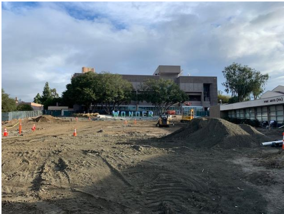
SC Fine Arts Quad Area – Nearing completion of Compaction
