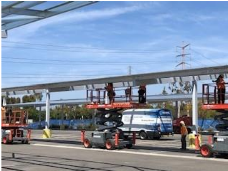
Electrical Connection between Modules
