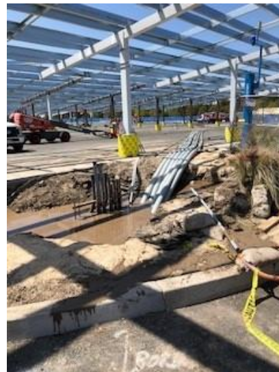
Underground Utility Boring
