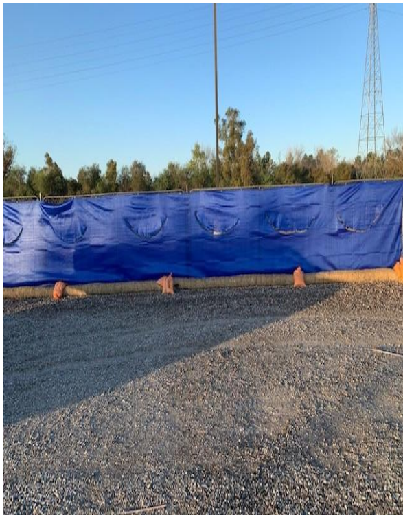
Temporary Chain Link Fence and Fabric
