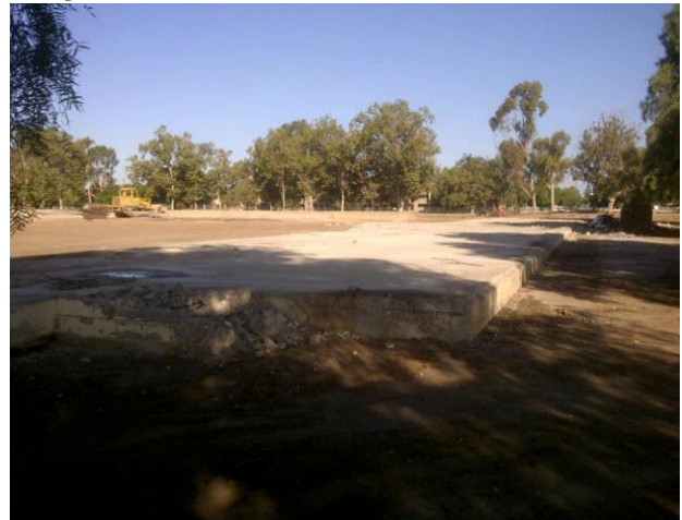
Building 134 – Slab Condition
