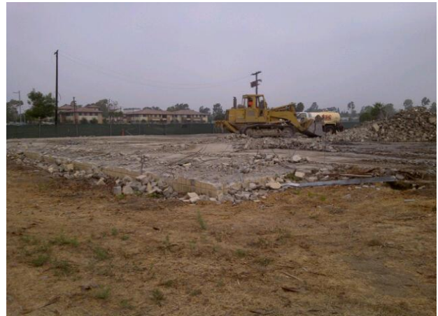
Bldg 166 – Slab Condition
