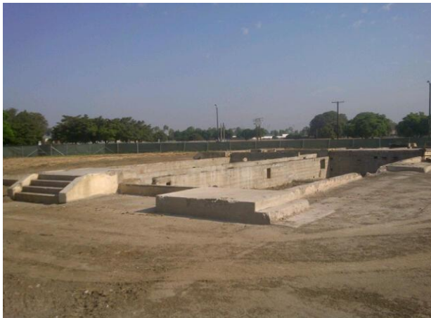
Bldg 4 – Slab Condition
