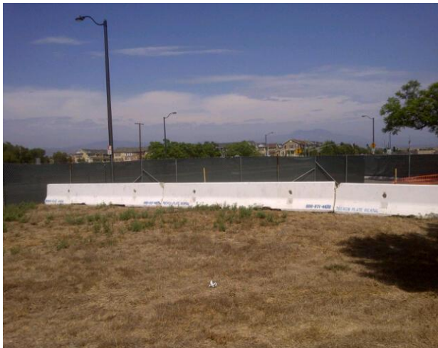
Demolition – K rail placement at Chapel Site
