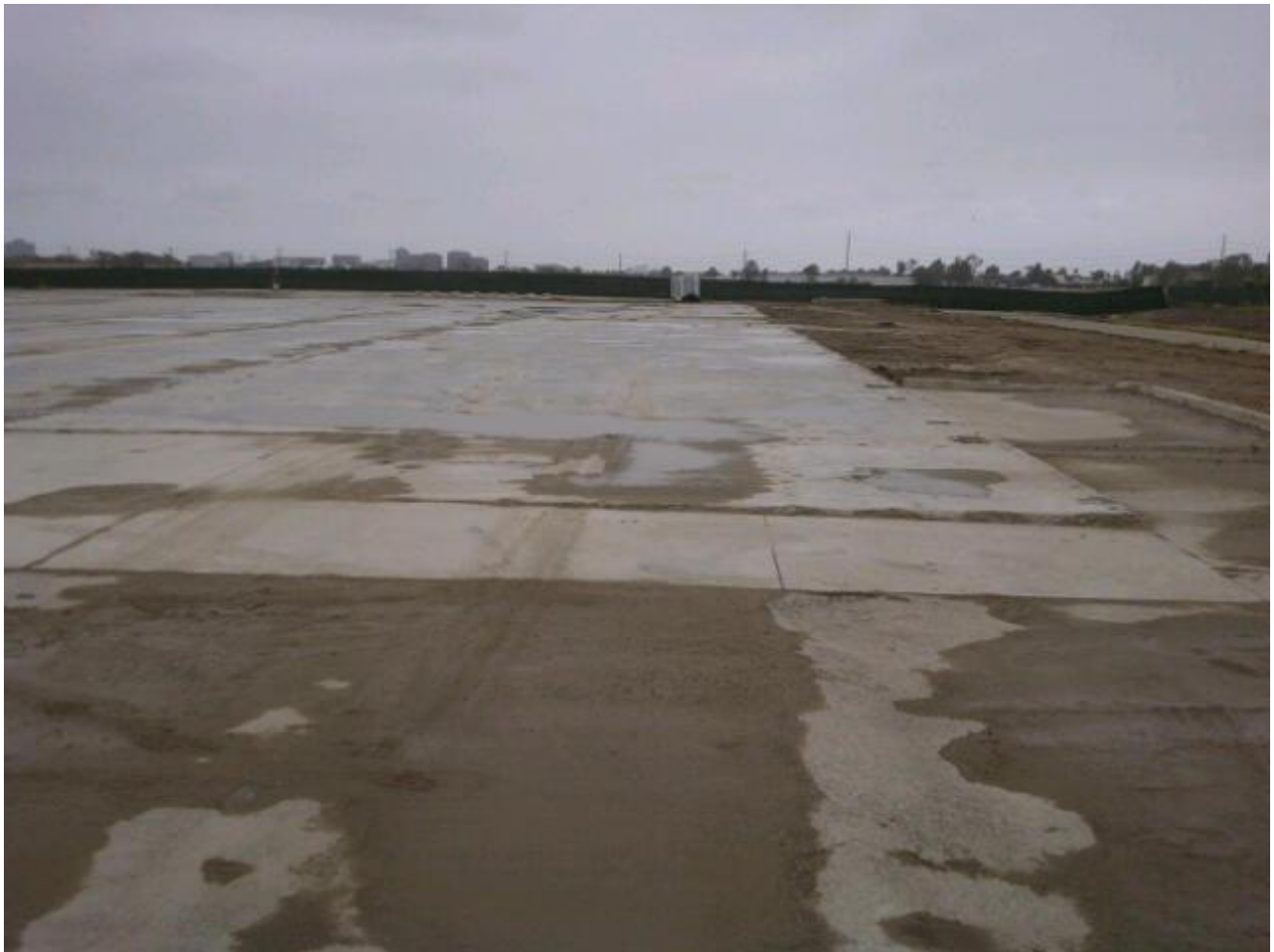
Demolition – Building 524 Slab Condition
