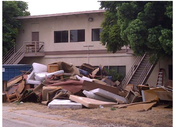
Bldg. 86 – Soft Demolition
