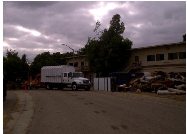
Bldg 86 – Soft Demolition and Tree Removal
