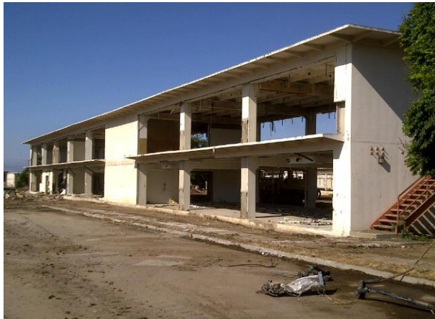
Bldg 88 – Soft Demo Completed
