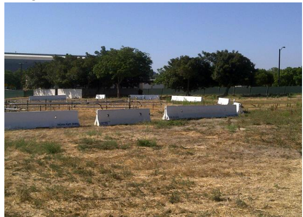
Parcel VI – K-Rail installation
