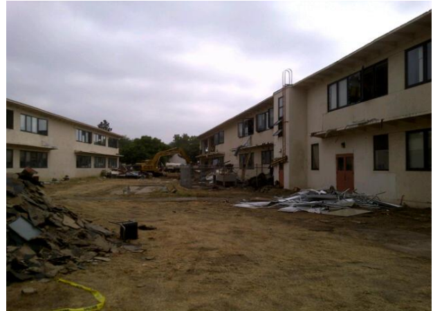
Bldg 87 & 88 – Soft Demolition
