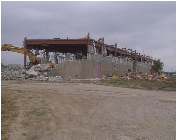
Demolition – Building 524 East Side
