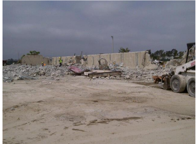
Demolition – Bldg 524 East Side
