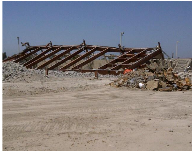
Demolition – Bldg 524 Southeast Side
