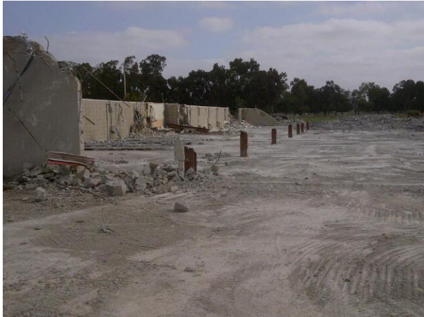
Demolition – Bldg 524 West Side
