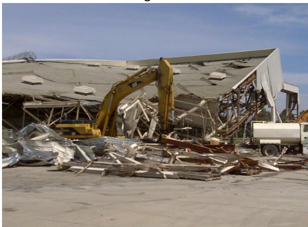
Demolition – Bldg 524 Southside
