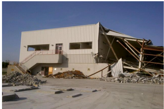
Demolition – Bldg 524 Westside
