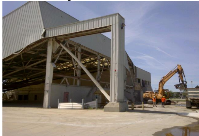
Demolition – Bldg 524 Eastside
