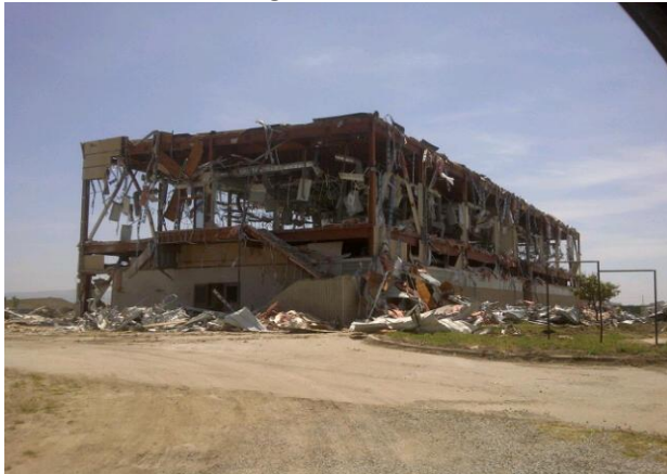
Demolition – Bldg. 524 Northeast Side
