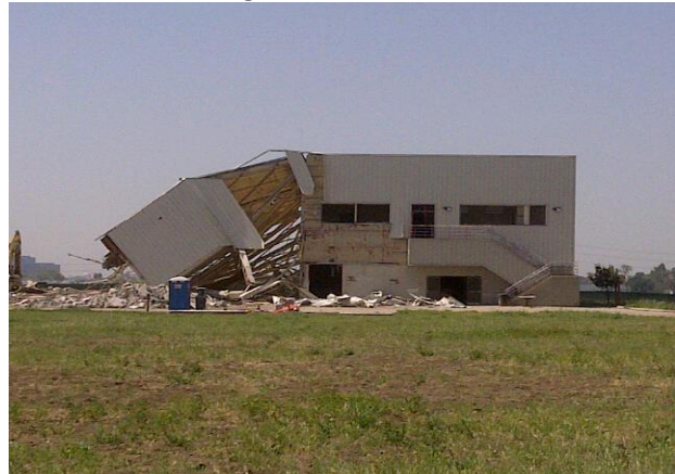
Demolition – Bldg. 524 East Side
