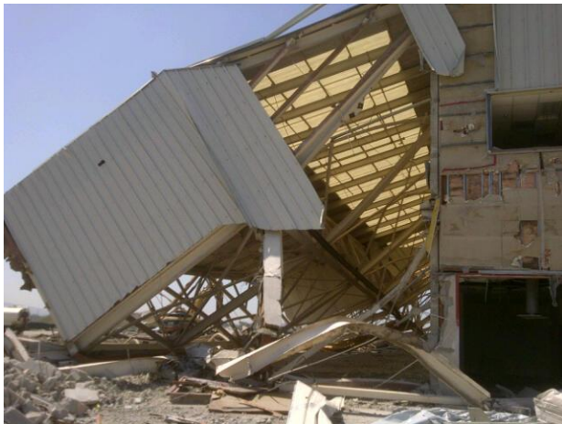
Demolition – Building 524 East Side
