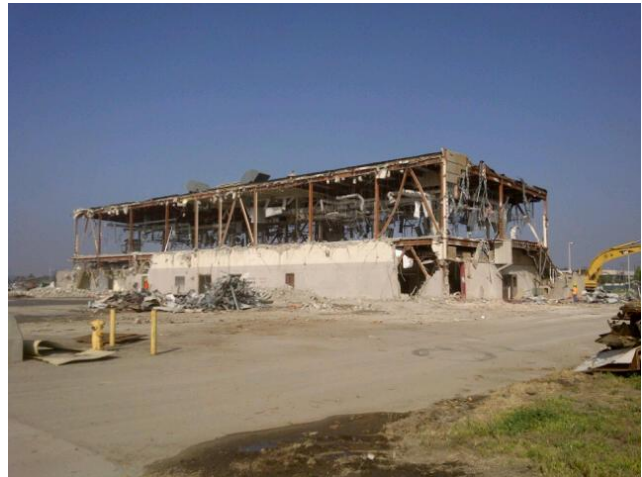
Demolition – Bldg. 524 Southeast Side
