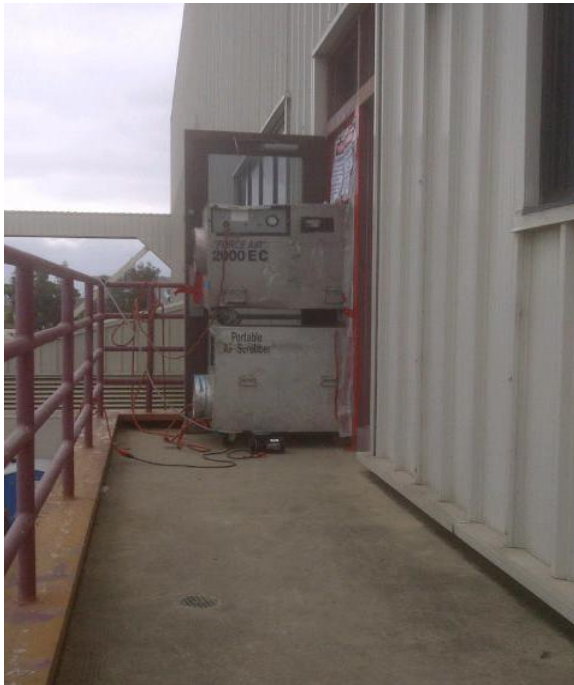
Abatement – 2 nd floor – Bldg 524
