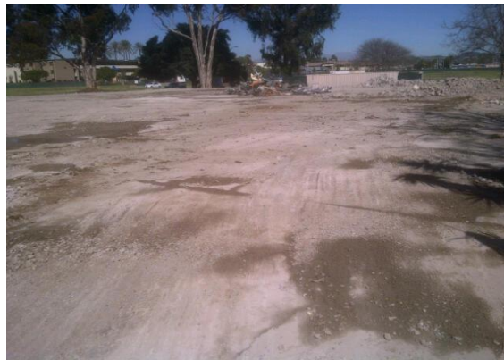
Bldg 184 - Slab Condition
