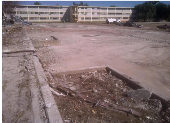
Bldg. 227 – Slab condition
