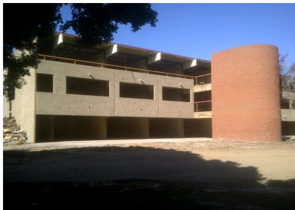
Bldg. 227 – Ready for Demolition
