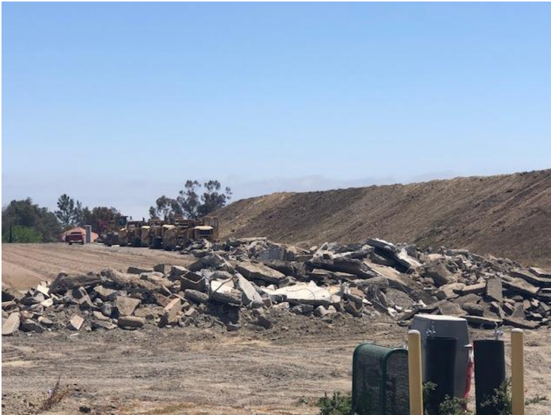
Contractor Demolishing Stadium and Stockpiling Concrete for Recycle
