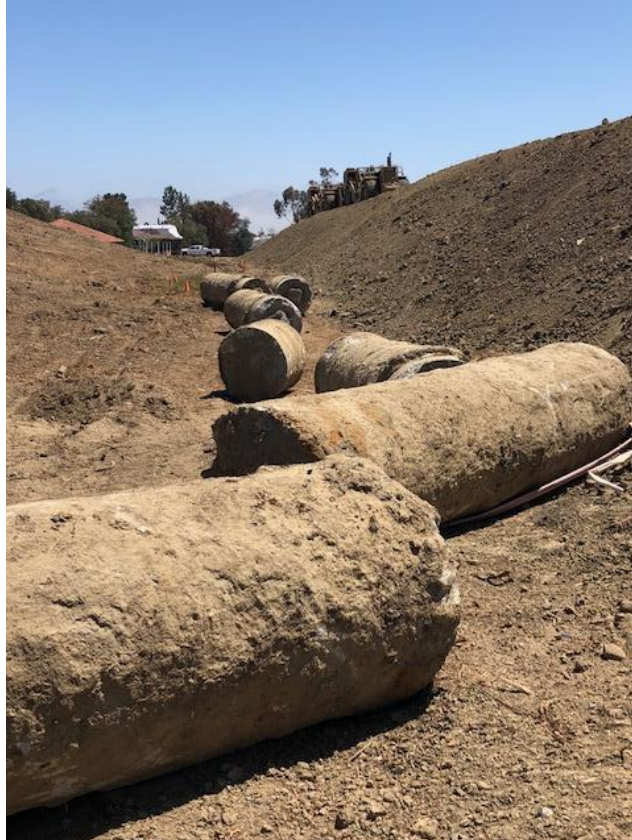
Demolition of Stadium Facility; Contractor Preparing for Earthwork and Grading
