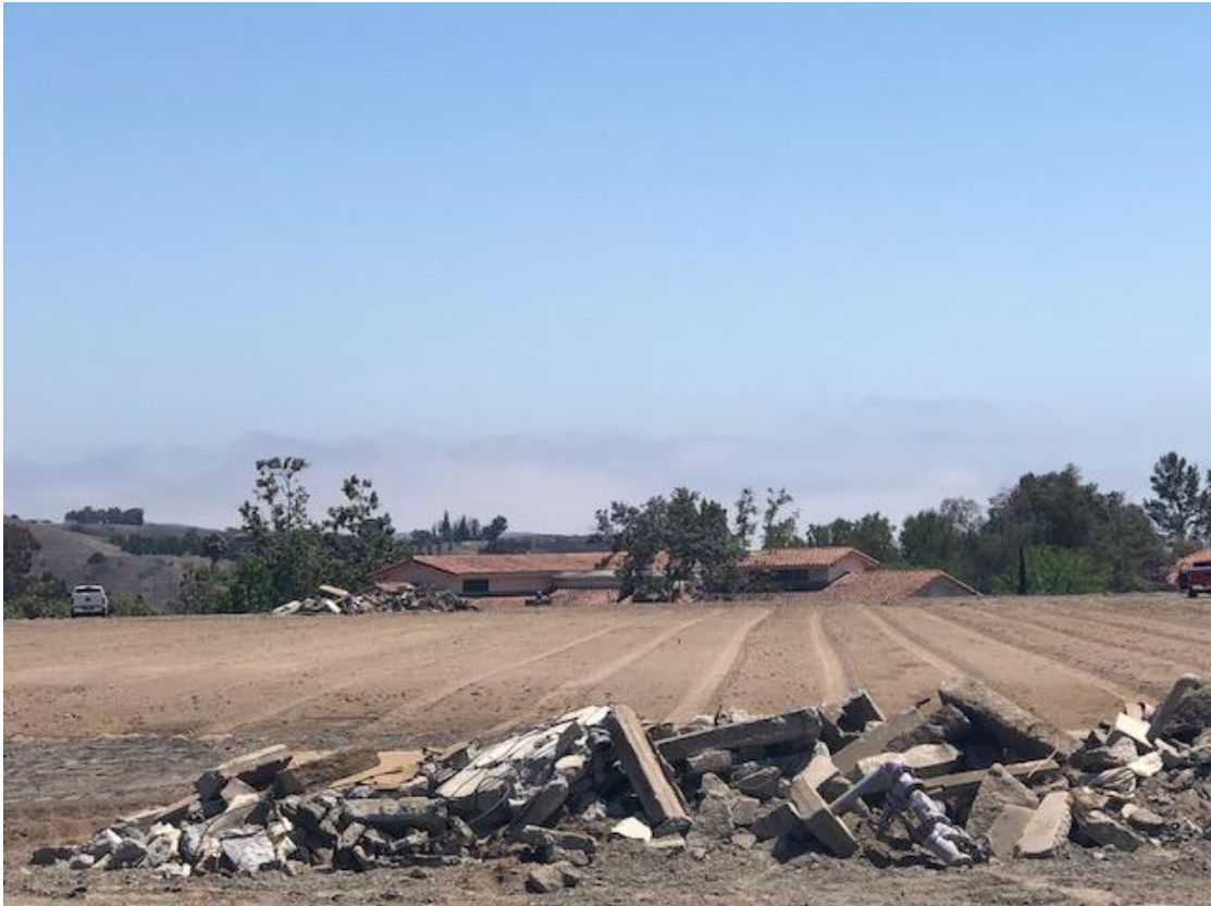
Demolition of Existing Stadium Facility
