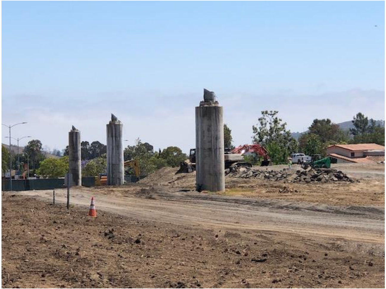
Contractor Demolition of Stadium Lighting Fixtures
